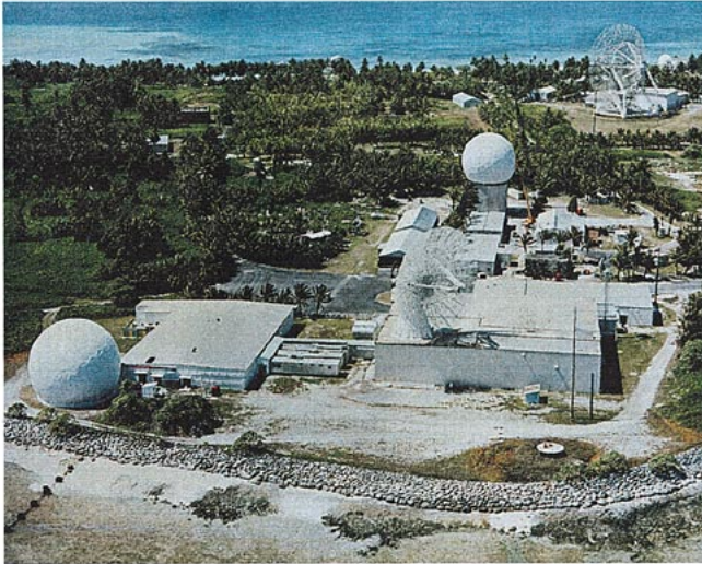
Fig. 3. The Kiernan reentry measurement system (KREMS) facility located on Kwajalein Atoll in the central Pacific Ocean. The ALCOR C-band radar is located under the white radome in the lower left of the photograph. The millimeter-wave radar is located under the smaller white radome near the center.
